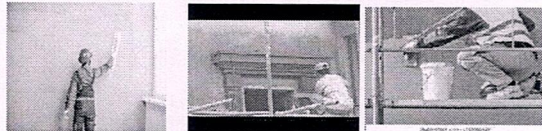
Inside Plastering 12mm Plastering 20mm
