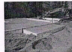
Back Filling with excavated earth and carted earth
